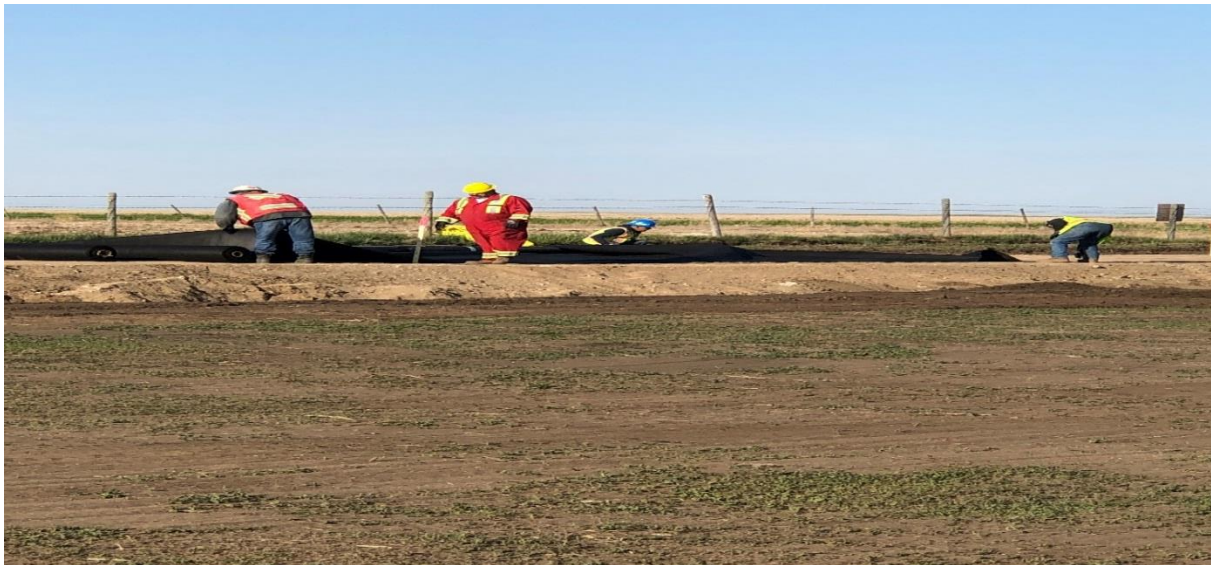
Crew laying Geo-Synthetic fabric along access road at MBLV 14.
