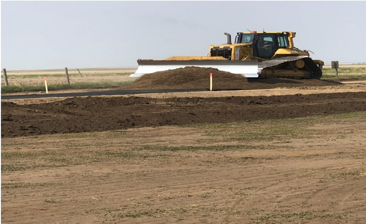
Spreading gravel along access road at MBLV 14.
