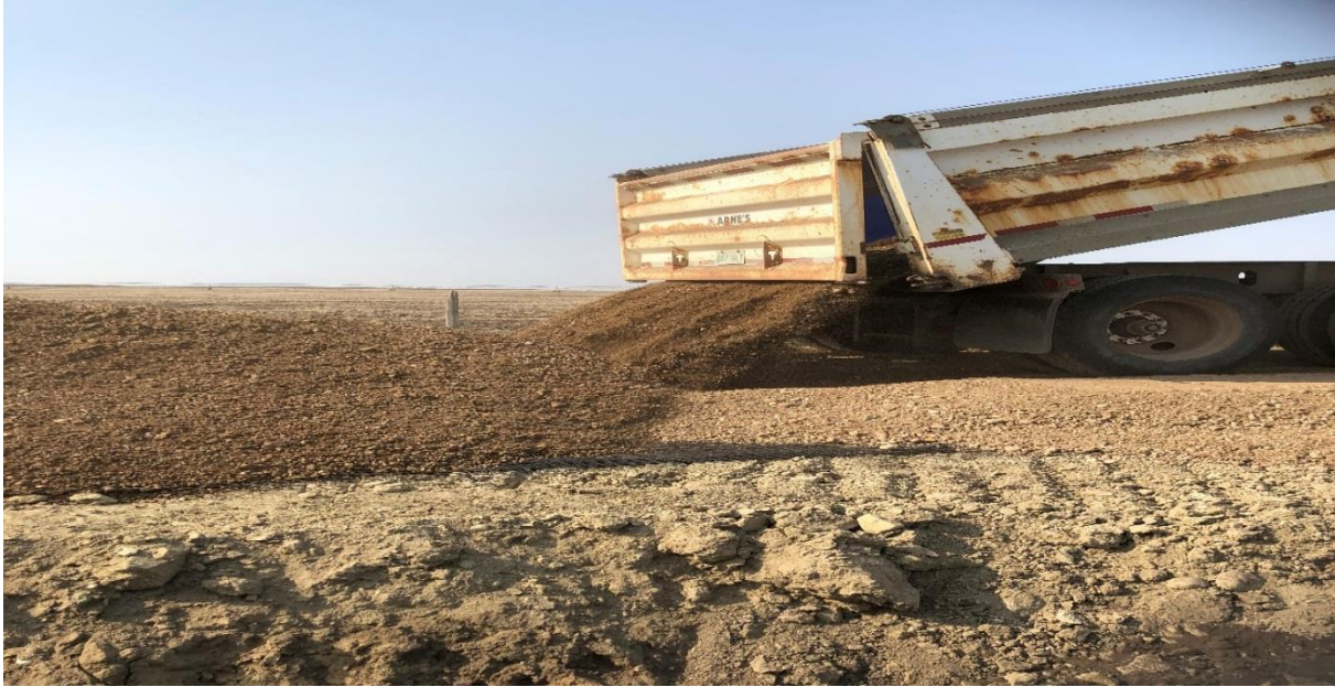
Unloading gravel atop access road at MBLV 14.
